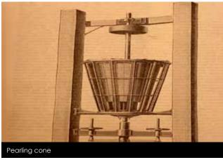
where the rice was polished by friction between the emery cement, which forms the working face of the cone and the wire covering of the outer case, the rice running through in a continuous stream.
